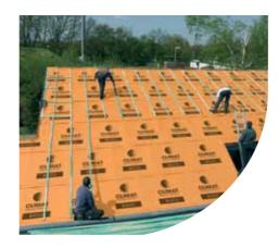
climat - Manufactured in Europe, this premium range of vapour-permeable roof and wall laminates uses Fiberweb's patented Linopore UV+ technology. Its exceptional heat and UV resistance makes CLIMAT ideal for use under solar panels and for building styles that might expose it to direct sunlight.
