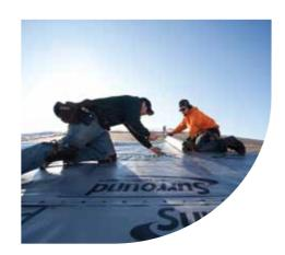
surround sr Roof Underlayment - The smart alternative to felt, SURROUND is lighter and quicker to install than roofing felt. Despite this, its waterproof polymer is strong, tearresistant and offers a safe, slip-resistant surface. One roll offers the same coverage as five rolls of standard roofing felt.
