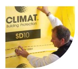
**CLIMAT X-Series** – Vapour-permeable roof underlays with Linopore UV+ and integrated adhesive strips to seal against water and wind.
