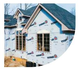
**TYPAR HouseWrap** - With exceptional air and water holdout, this material provides comfort and energy efficiency while controlling moisture intrusion. TYPAR Weather Resistant Barriers hold back air and moisture from the outside while allowing moisture vapour to escape from inside.
